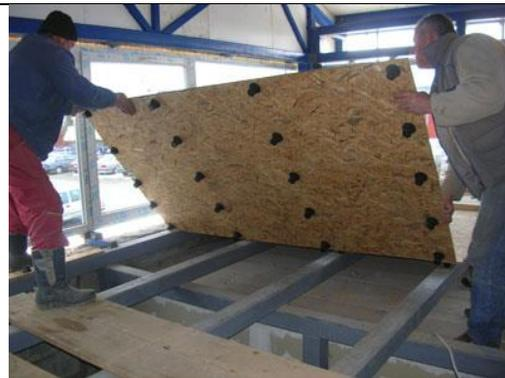
8. Incorporating revision holes in the floor, we get the opportunity to control or retrofitted wiring, as well as performing pest and rodent control.
